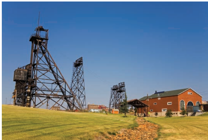
FIGURE 4.2 Underground mine head frame and hoist room. SOURCE: Photograph courtesy Richard Cummins/SuperStock.
