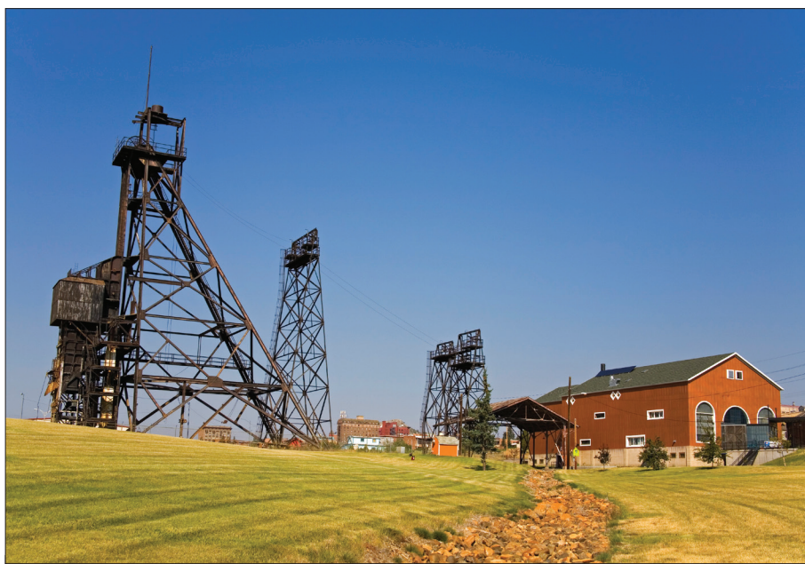
Figure 5. Underground mine head frame and hoist room.
