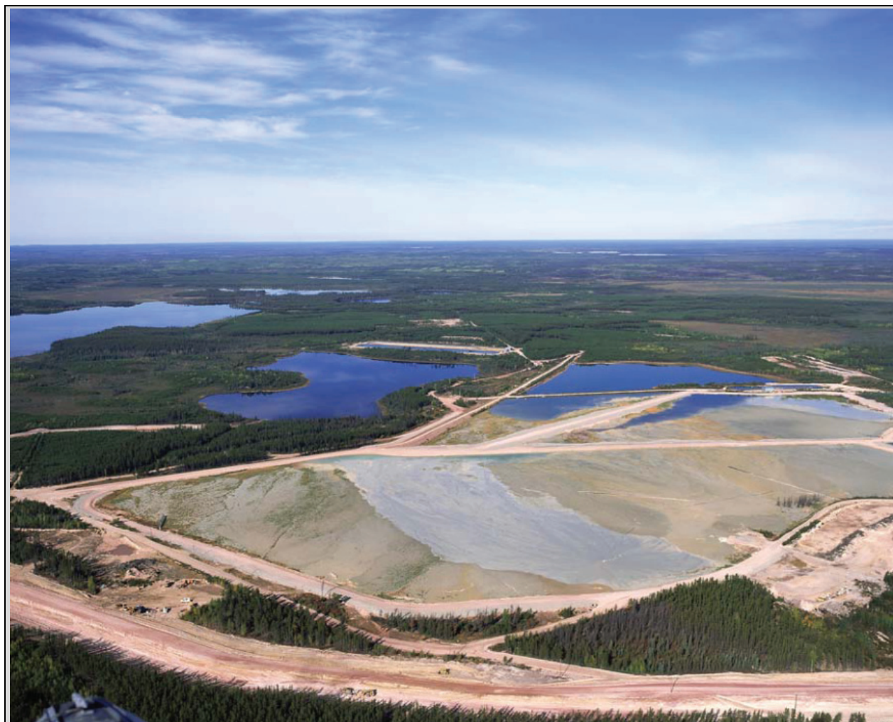
FIGURE 6.1 Tailings management area at Cluff Lake in 1999, Saskatchewan, Canada. The tailings are held behind an earthen dam. SOURCE: AREVA Resources Canada Inc.
